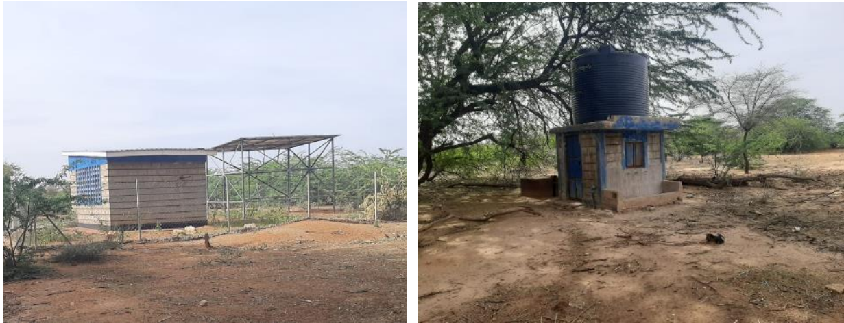
Plate 2: Sereolipi Water project
